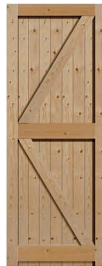
FIG. 44 LEDGED, BRACED AND BATTENED DOOR
